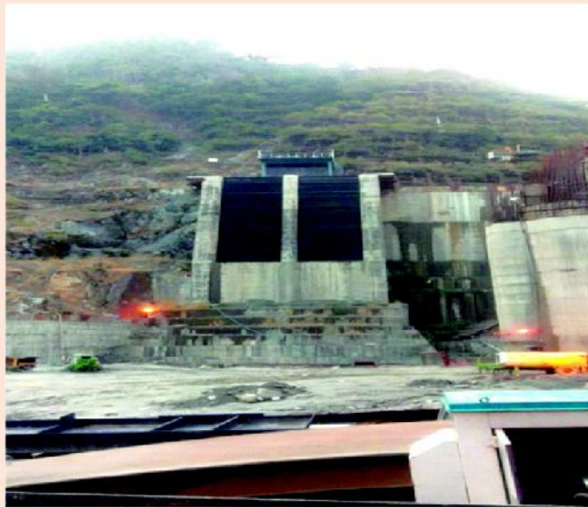
Intake Gate, Trash Rack Panel, Hoist Arrangement
