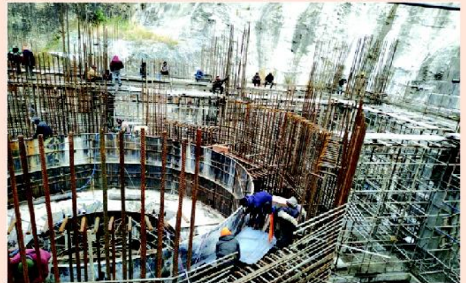
Unit 2 power house shuttering and reinforcement in progress
