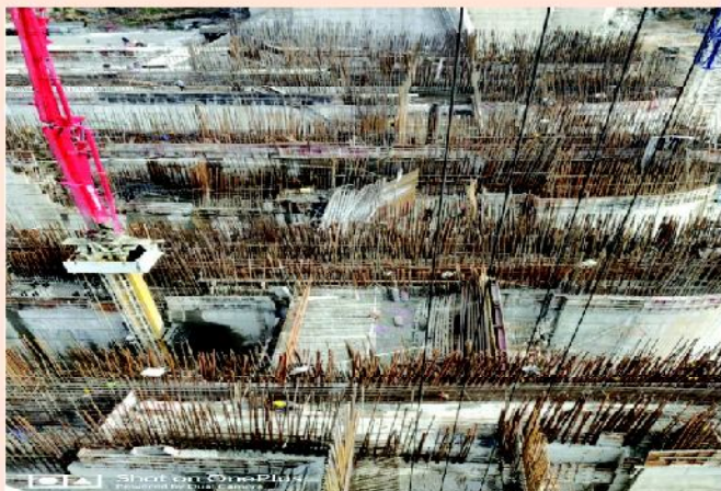
Dam Overflow Blocks
