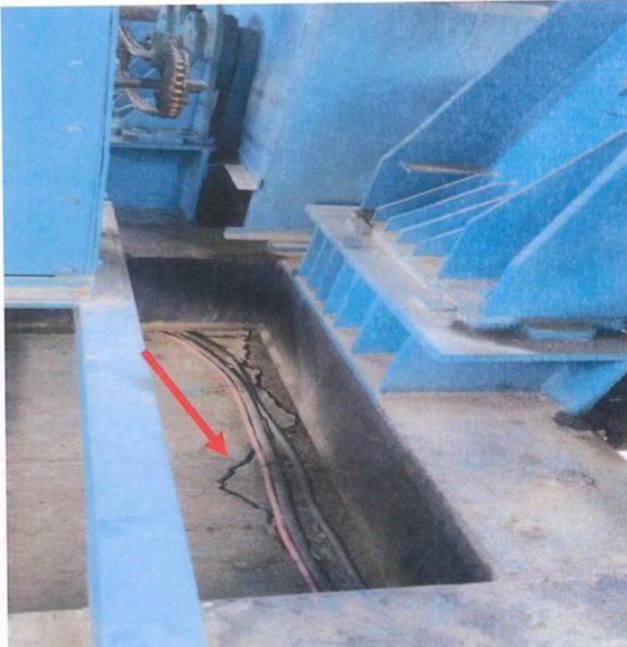
Crack at top left abutment of barrage near hoist
