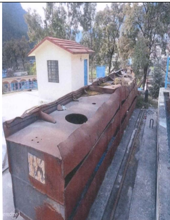
Damaged stop log gate
