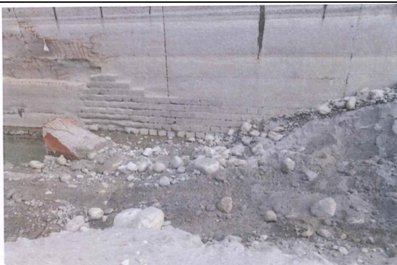
Damaged EDA area at d/s of Joshiyara barrage
