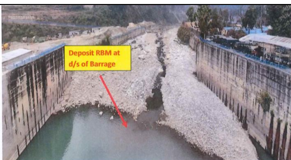
Accumulated RBM at d/s of Joshiyara barrage
