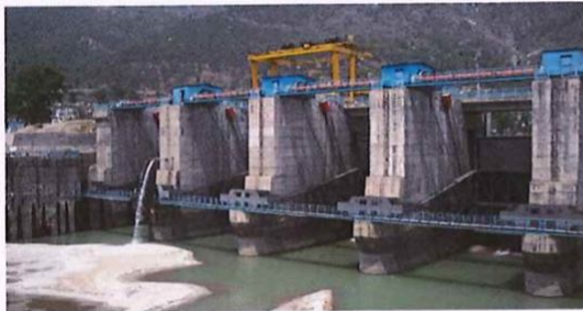
Radial Gate Barrage
