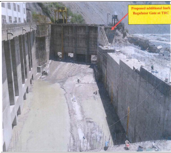
Construction/provision of additional back regulator TRC gates at Dharasu power house site
