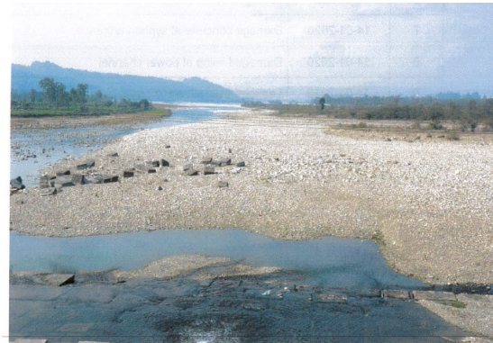
Eroded Apron on Barrage
