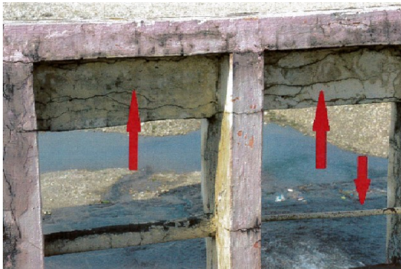
Damaged railing Barrage
