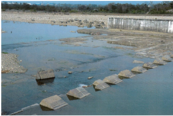
Damage Energy Dissipation System of Asan Barrage
