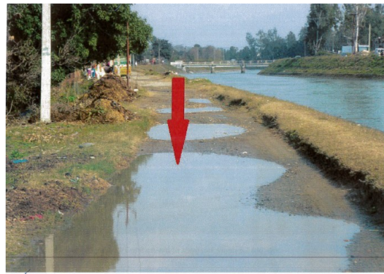
Damaged service road on right bank of power channel
