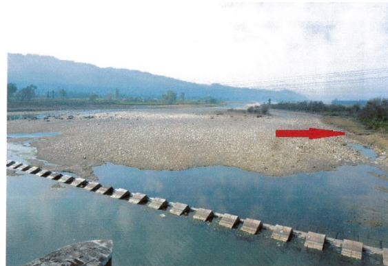
Silt deposit in Front of bay on 8 to 14 down steam of barrage
