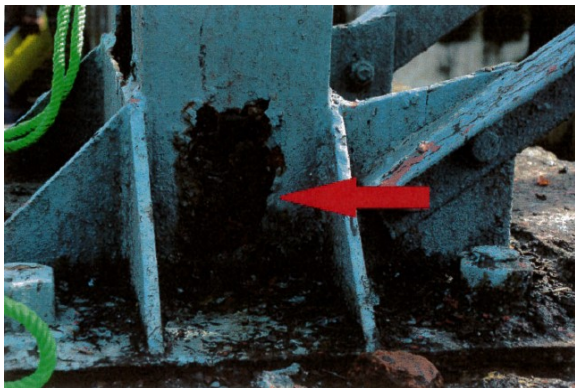
Damaged shoe of hoist bridge column of HR
